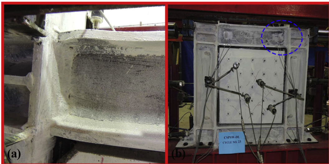
Fig. 11. The inelastic buckling of the upper beam flange of specimen C-SPSW-DL in 3.36% drift: (a) front view (b) back view.
